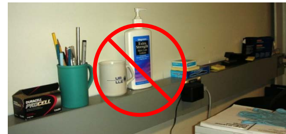
Raceway storage NOT OK
