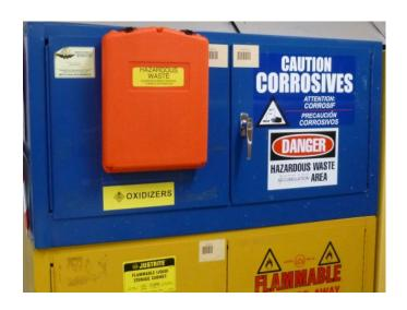
Accumulation start date labels are located in the red-box in the Hazardous Waste accumulation area
