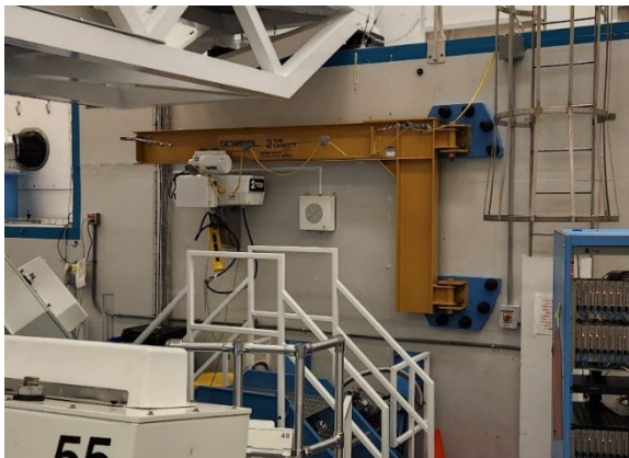
Wall Mounted Jib Crane (East side, Omega)
