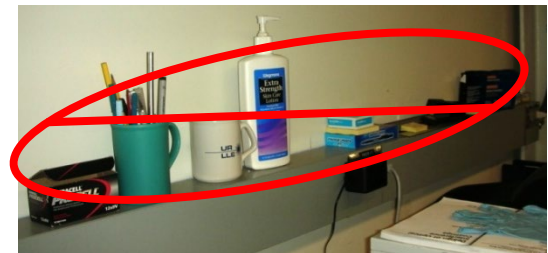
Raceway storage NOT OK
