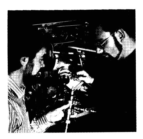
Roger Gram, Research Engineer, and Mark Wittman, Senior Technical Associate, prepare polymer-shell targets for sputter-coating with aluminum. A thin aluminum layer significantly increases the retention time for gases, while remaining sufficiently transparent to allow interferometric measurement of gas content. These shells would otherwise be much too permeable to retain gases long enough to conduct ICF experiments.
