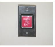
To exit LaCave after the doors have been locked, you must press and <u>HOLD</u> the illuminated square button while opening the door.
