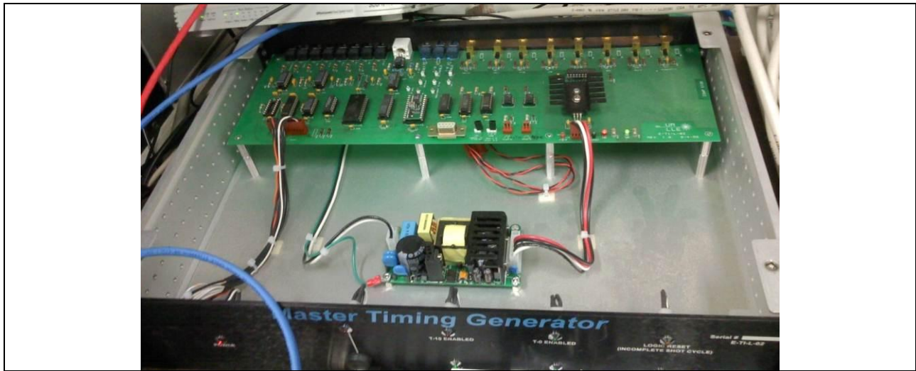
Fig. 3 Old MTG, internal view: Obsolete components and a sparse readout.
