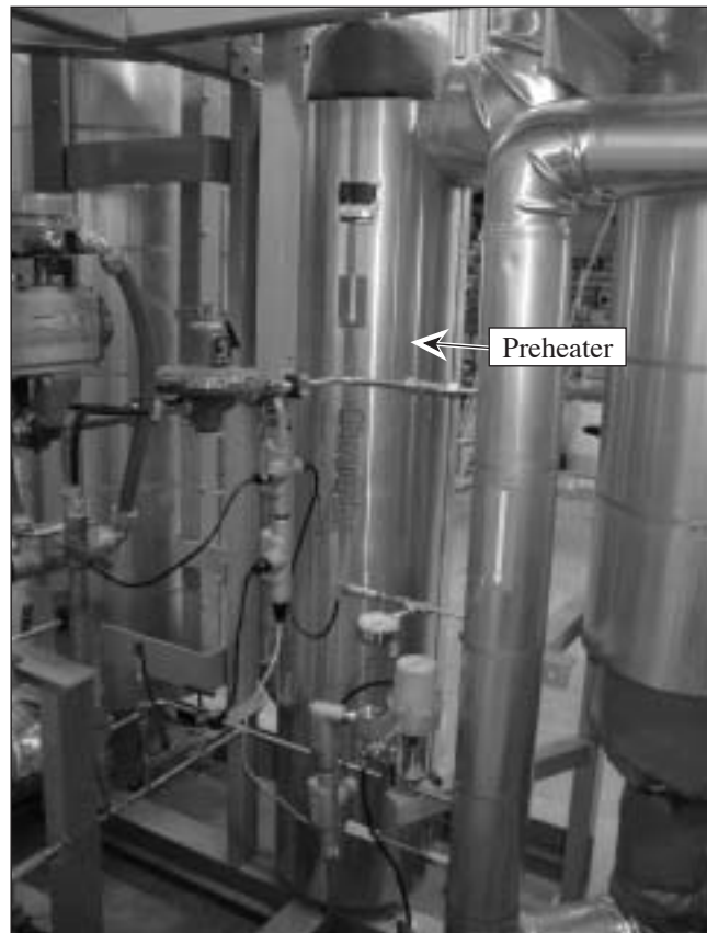
Figure 12.2-7 Reactor preheater.
