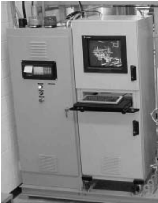
Figure 12.4-1 The operator workstation, PLC, and PC cabinets.
